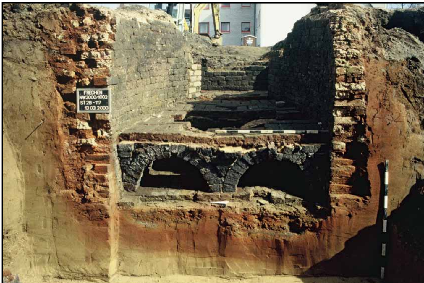
Abb. 55 Mixed cross-draught / down-draught earthenware kiln with a raised kiln floor on a double archway. Frechen, Nordrhein-Westfalen D, Alte Straße 67–73 (Foto Cornelius Ulbert, archaeologie.de).
